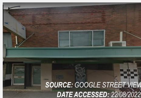
FIGURE 6: VIEW OF 318 KINGS GEORGE ROAD ADJOINING TO THE EAST
