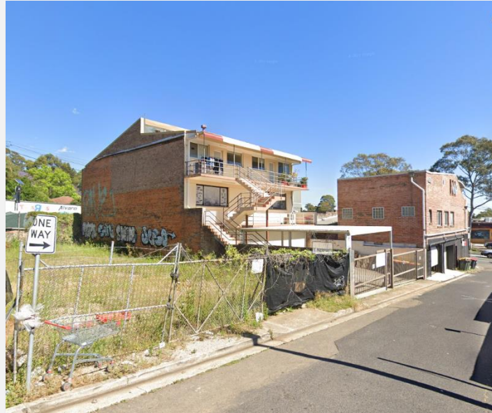
FIGURE 13: PROPERTY 306-308 KING GEORGES ROAD DEMONSTRATING ELEVATED 2 STOREY APPEARANCE.
